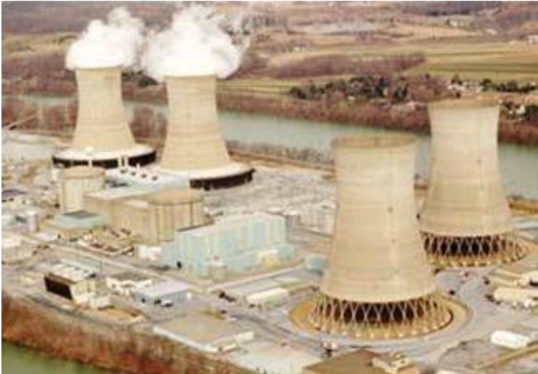
Nuclear Power Station
